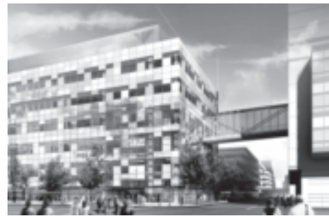
Barry Svigals, Yale-New Haven Hospital, with Behnisch Architects.
