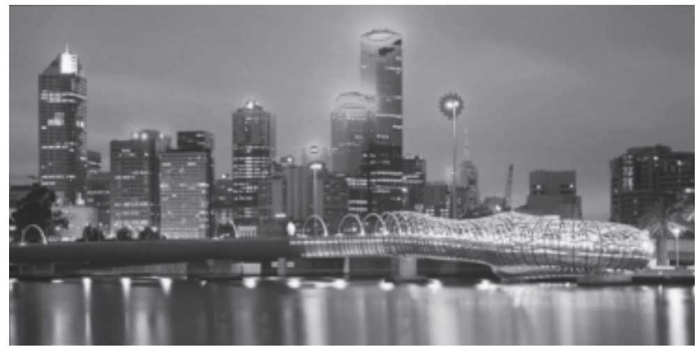
Denton Corker Marshall, Webb Bridge Melbourne, 2006. Courtesy Critical Visions 08.
