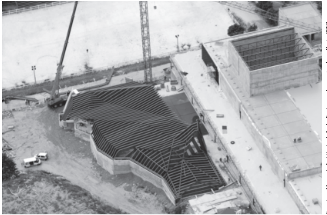
Francisco Mangado Architects, Avila Auditorium under construction, Spain, 2007.
