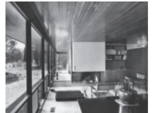
Joeb Moore, renovation and restoration of the Glenn Residence, Stamford, Connecticut, by Richard Neutra.
