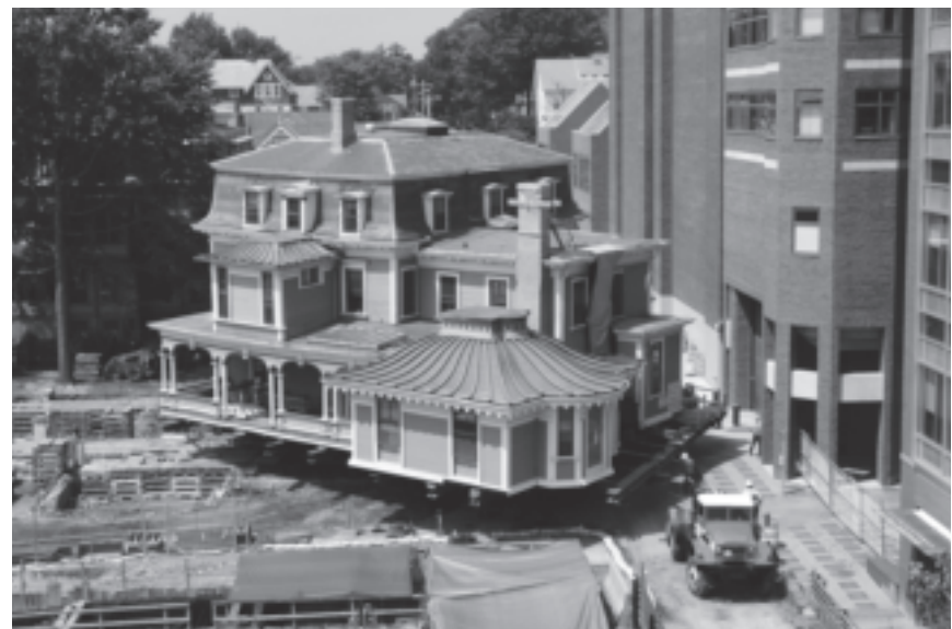
Kliment Halsband Architects, Peter Green House being moved at Brown University, summer 2007.
