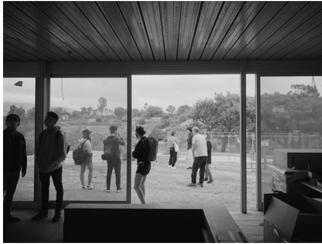
Taalman Architecture, Malibu IT House, Malibu, under construction, photograph by Daisy Ames, 2021
