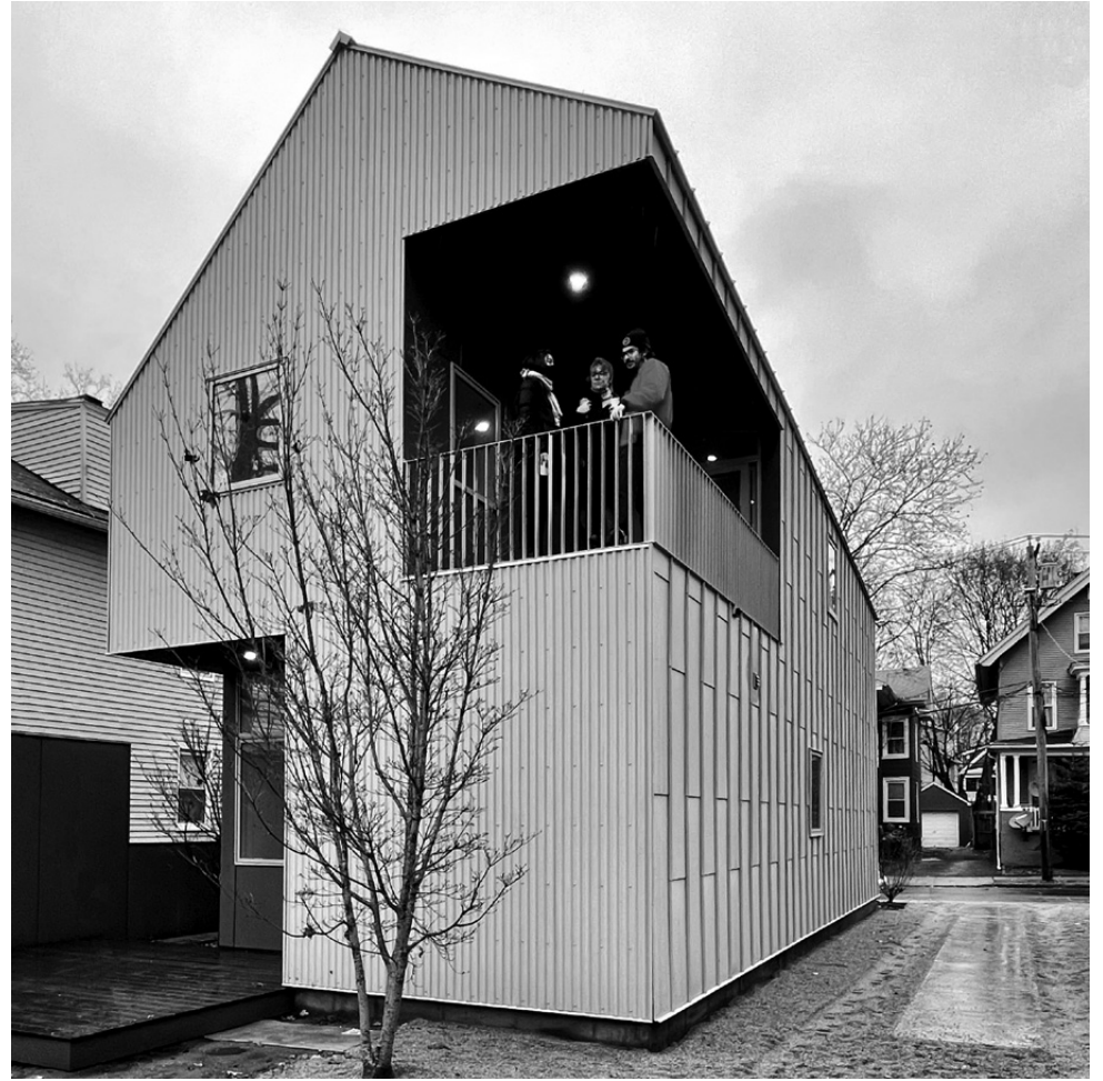
2021 Yale Building Project with Columbus House, photograph by Alex Kruhly
