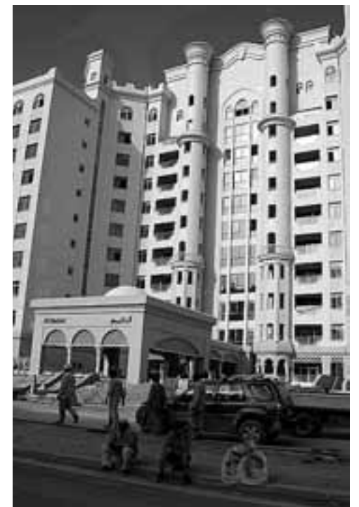
New building with "traditional" elements Photograph by Elisa Lui, Ali Rahim's studio trip, spring 2007.
