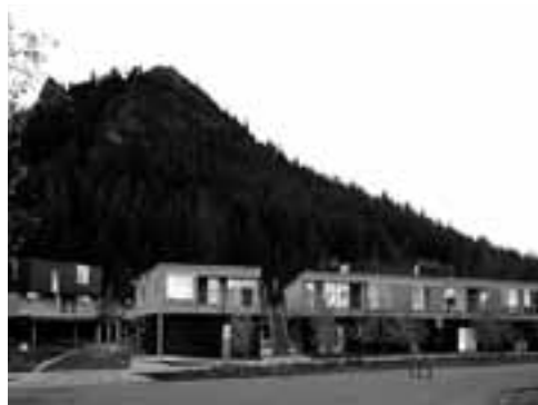
Peter L. Gluck & Partners Architects, Little Ajax Affordable Housing, Aspen, Colorado, 2007.
