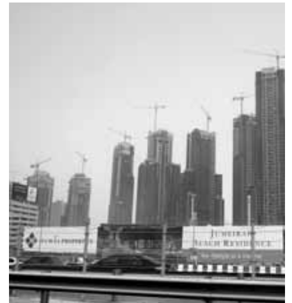
Dubai construction process. Photograph by Elisa Lui, Ali Rahim's studio, spring 2007.
