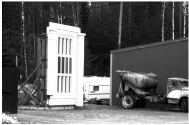
A concrete element for Arc at Södra Station by Ricardo Bofill, Stockholm, ca 1989, courtesy Jan Inghe-Hagströms arkiv, Stockholm City Archive
