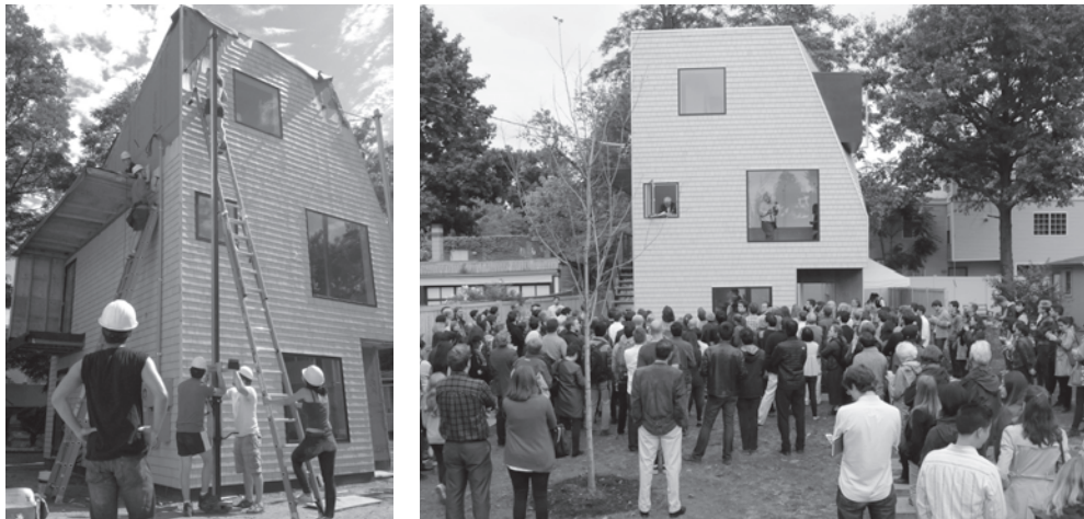
Jim Vlock Building Project, New Haven, 2014.
