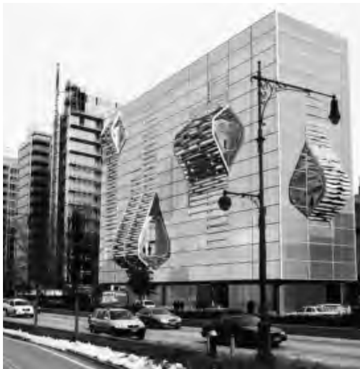
Servo, rendering/montage of a hypothetical site for the distribution of Lobbi-Ports in an existing residential building on the West Side of Manhattan.
