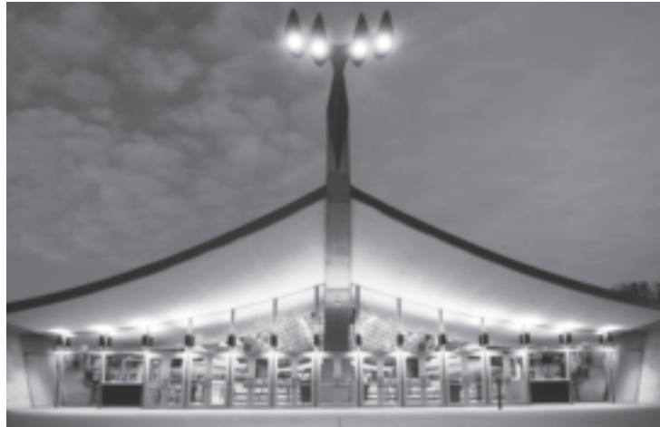
Eero Saarinen, Ingalls Rink (1958), Yale University, New Haven, restoration by Kevin Roche, 2009. Photograph by Michael Marsland, 2009.
