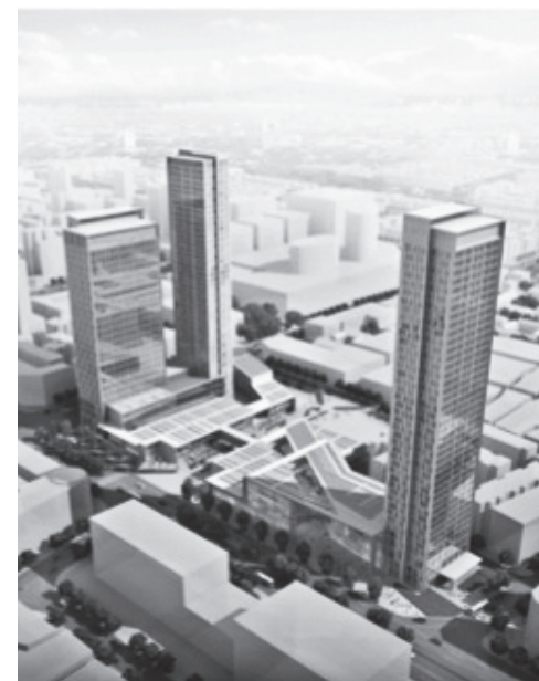
Tishman Speyer, Eco-City, Skidmore, Owings & Merrill, Chengdu, China.
