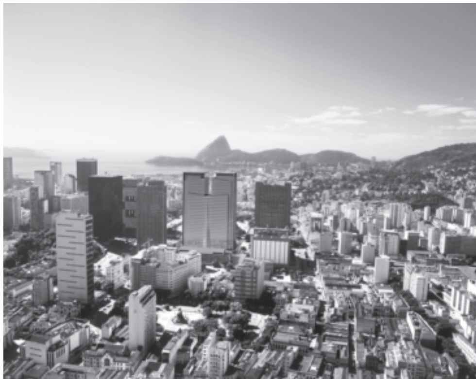
Tishman Speyer, Ventura Towers, Kohn Pederson Fox/ AKGV Architects, Rio de Janeiro, Brazil.
