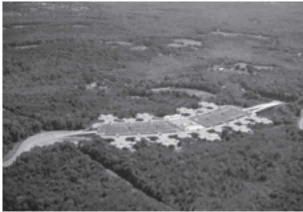
KRJDA, Union Carbide Corporation World Headquarters, Danbury, Connecticut, aerial view, 1976–82.
