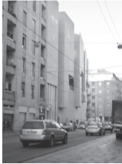
Grafton Architects, Luigi Bocconi University, view from Viale Bligny, Milan, 2008.
