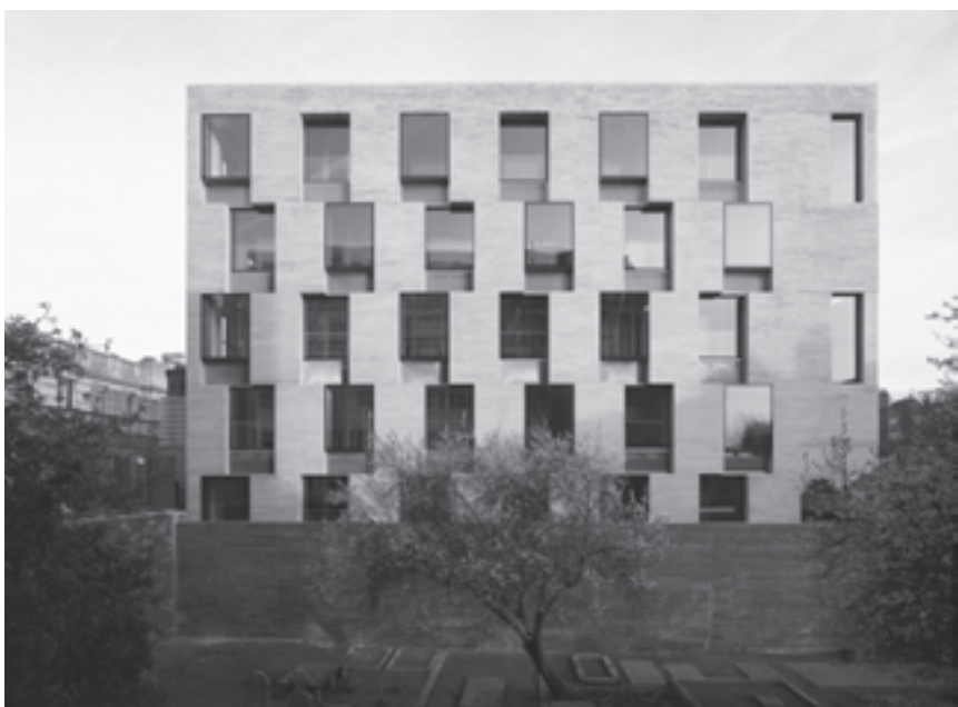
Grafton Architects, 7-9 Merrion Row + The Billets, Department of Finance Offices, stone façade to Huguenot Cemetery, Dublin, 2008. Photograph by Dennis Gilbert.
