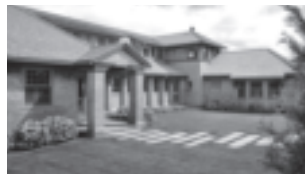
Albert, Righter & Tittmann Architects, Island Cove, Martha's Vineyard, 2021, photograph by Robert Benson
