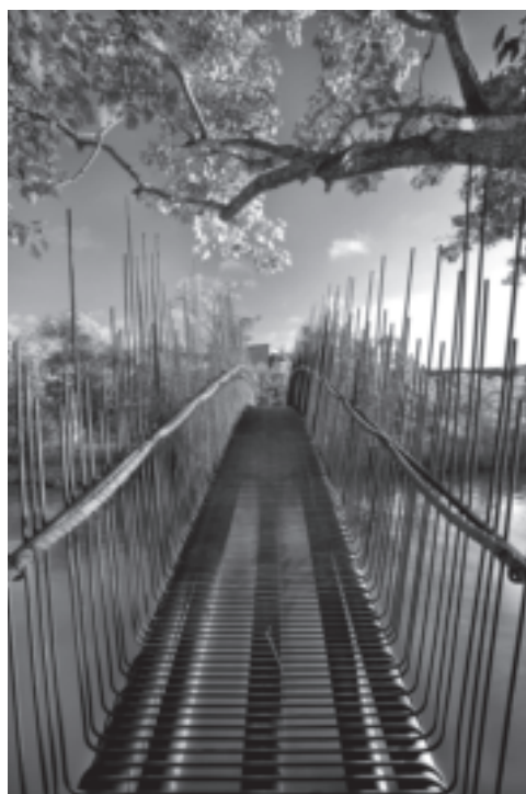
Miro Rivera Architects, Pedestrian Bridge, Austin, Texas, 2007, photograph by Paul Finkel, Piston Design.
