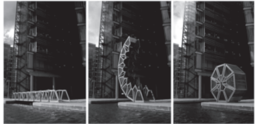
Rolling Bridge, London, Thomas Heatherwick Studio, photograph by Steve Speller, 2003.
