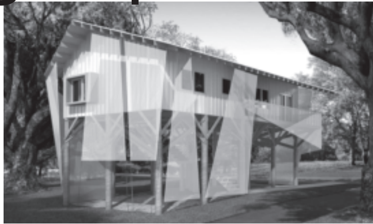
Bryan Bell, Design Corps, Biloxi project in progress, 2007.
