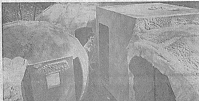
Rooms of houses follow contour of plastic-backed burlap balloons. A cubo varies this design.
