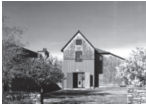
Albert, Richter & Tittmann Architects, Geothermal House & Barn, Hudson River Valley, photograph courtesy of Albert, Richter & Tittmann Architects, 2008.
