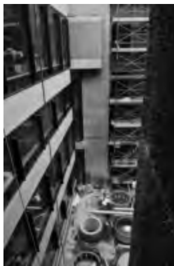
Restoration of Paul Rudolph Hall in process, spring 2008.
