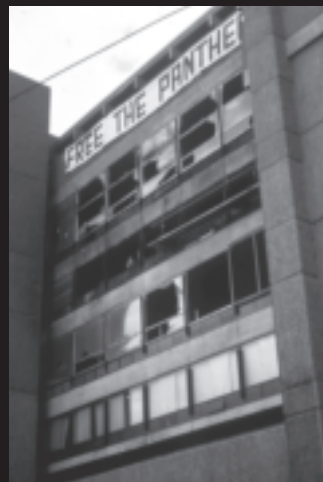
The Art & Architecture Building after the fire in 1969. Photograph by James Righter, courtesy Yale University Library, Manuscripts & Archives.
