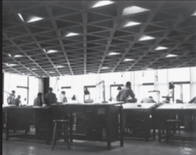
Drafting room on the fourth floor of the Yale University Art Gallery and Design Center, c. 1953. Courtesy Manuscripts & Archives, Yale University
