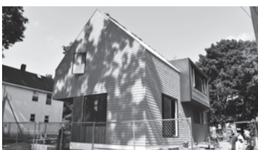
Jim Vlock Building Project 2018 under construction, photograph by Deo Dieparine ('20)
